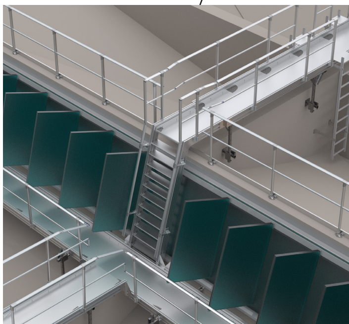
Intersection between step ladder, gangway and stairs.
